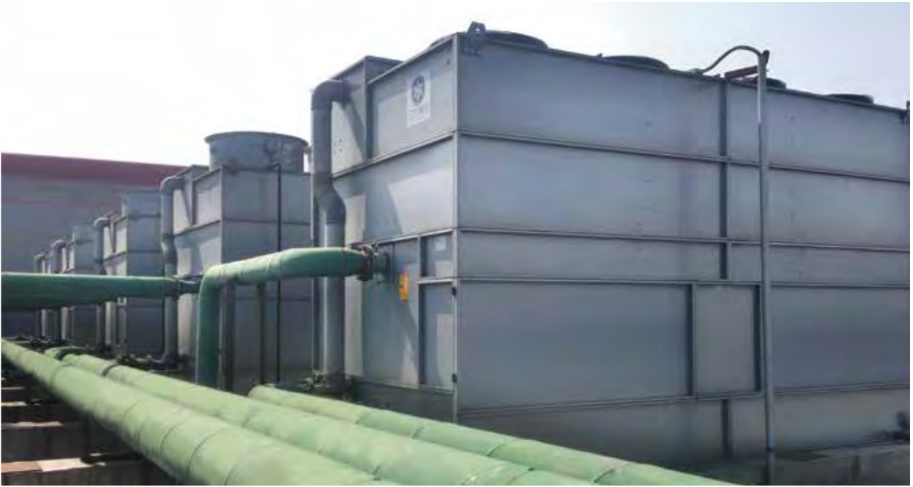
◆ For SiDa MF. Induction Furnace
