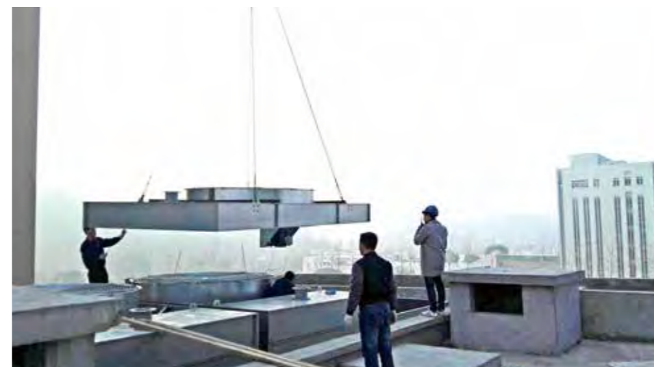
Fabricating at Project Site
